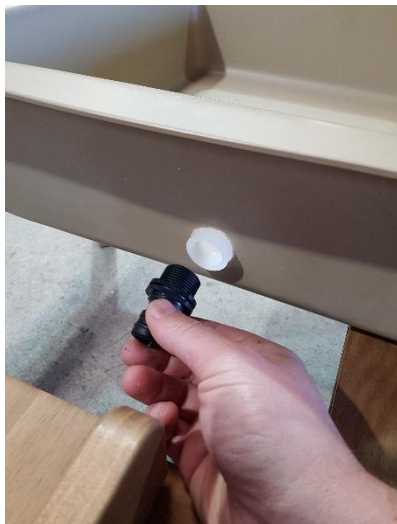
Screw the threaded male fitting into the tub.
