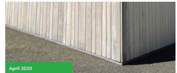
Cladding project, North America
